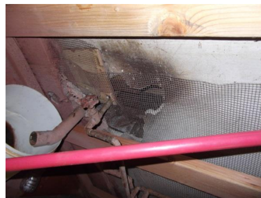
Illegal installation of grease trap
