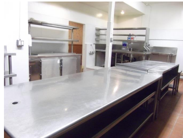
Elimination of rodent entry points
